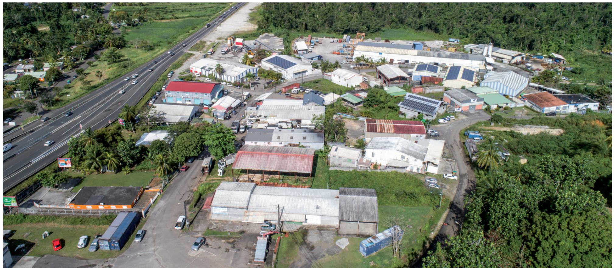
ZAE de Beausoleil, Baie-Mahault
